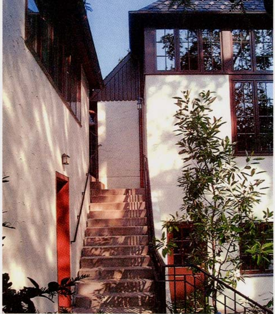
Stairs to the upper courtyard make a natural transition between the two buildings.
